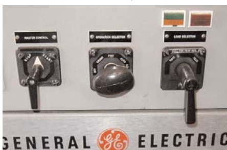
Clockwise from top Figure 2: Operation selector switch in remote start position at base load
