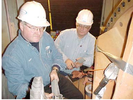
Charlie Pond and Skip Beck change first-stage turbine buckets
