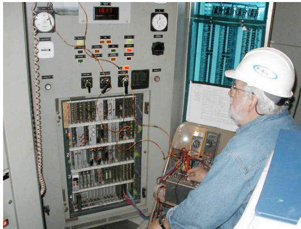
Dave Lucier Calibrating Speedtronic™ Mark I panel at Ameren-UE, Jefferson City, MO
