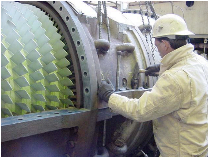
Millwright installing dowels on a compressor casing
