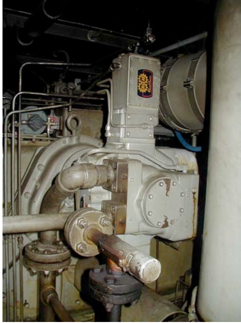
Fig. 1- OilGear Fuel Pump
