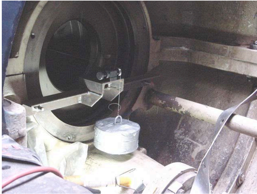
30-pound weight ensures correct wire sag; fixture sets proper wire position
