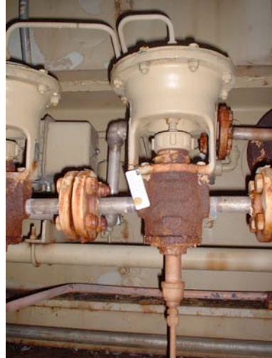
Fig. 1: Some typical VA19-1 liquid fuel purge valves
