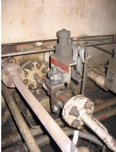
Fig. 1: Some typical VA19-1 liquid fuel purge valves
