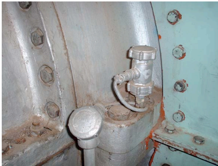
Fig. 2: Vertically mounted Velocity (seismic) Pickup
