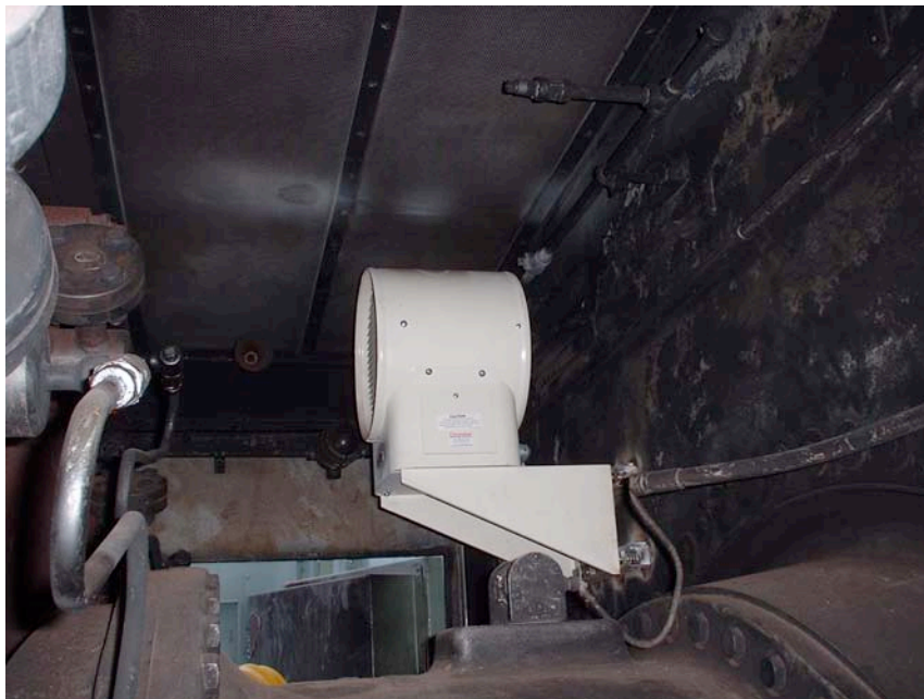
Fig. 1: Typical Turbine Compartment Heater
