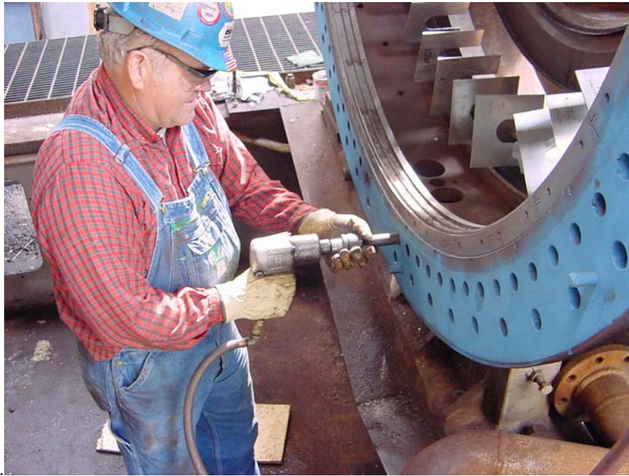
CLEANING THE COOLING AIR PASSAGES
