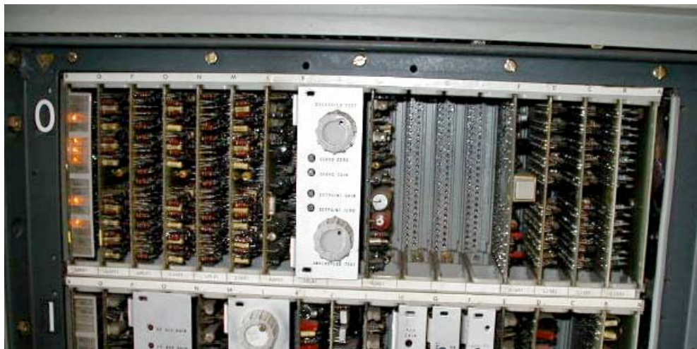
Fig. 7: Spare Locations for LINA cards in Row 0 (Slots F, G & H) on Speedtronic Panel
