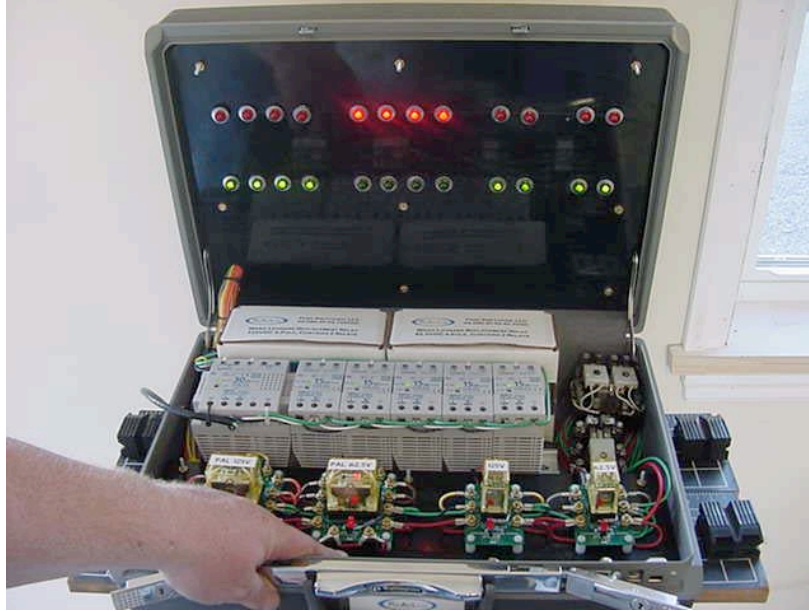
Fig. 2: 4-pole PAL relay being tested showing contact closures with red LED
