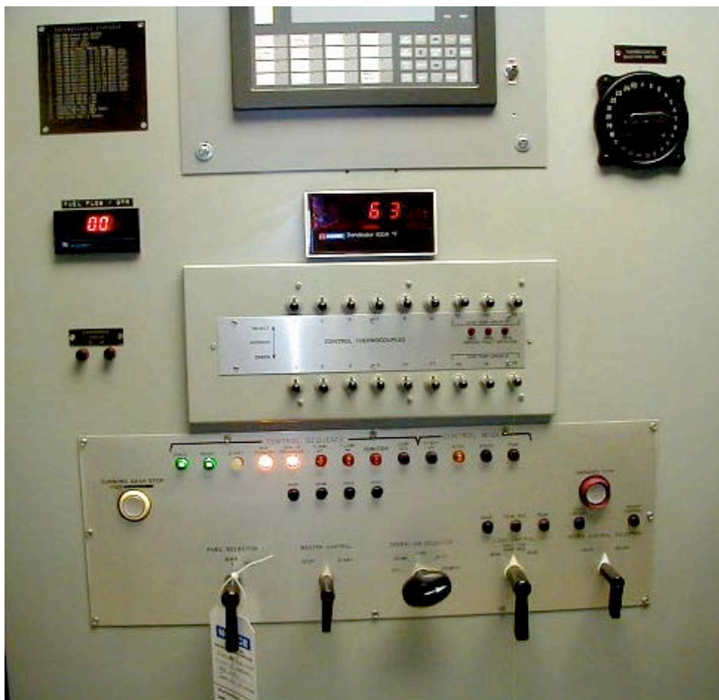
Fig. 3: After-market flow meter shown in upper left hand corner of the photo above
