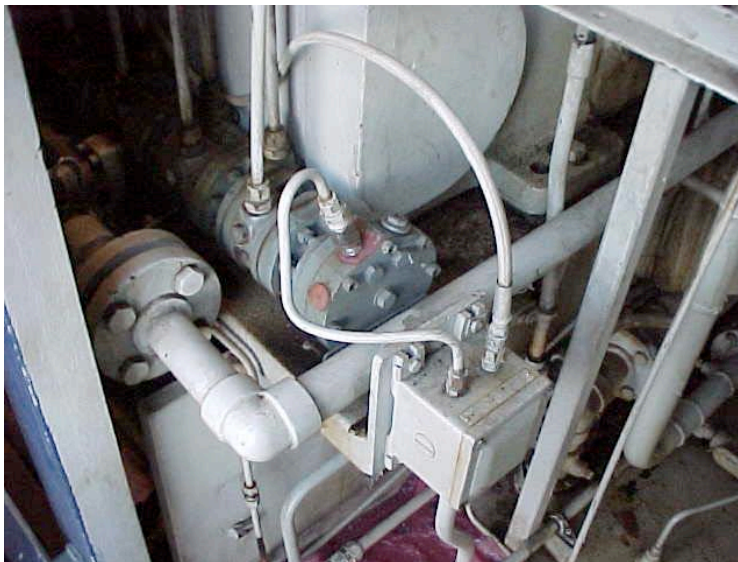
Fig. 2: Roper flow divider with one speed pickup on right end
