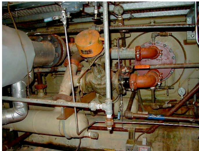
Fig. 5: Robertshaw Temperature Regulator Valve, VPR
