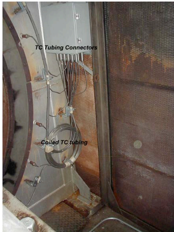
Fig. 2: Thermocouple tubing leads coiled and run up to the "pass through" box.
