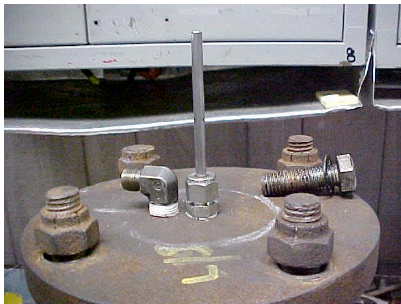
Fig. 5: "Tell Tale" Indicator Rod emerging from the top of the Recirculation Valve
