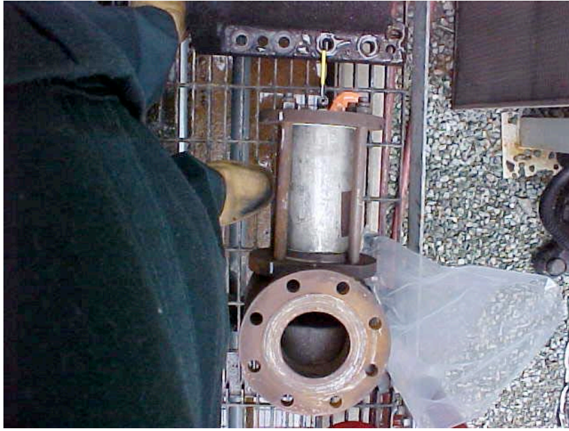
Fig. 5: Valve ready for re-installation on compressor
