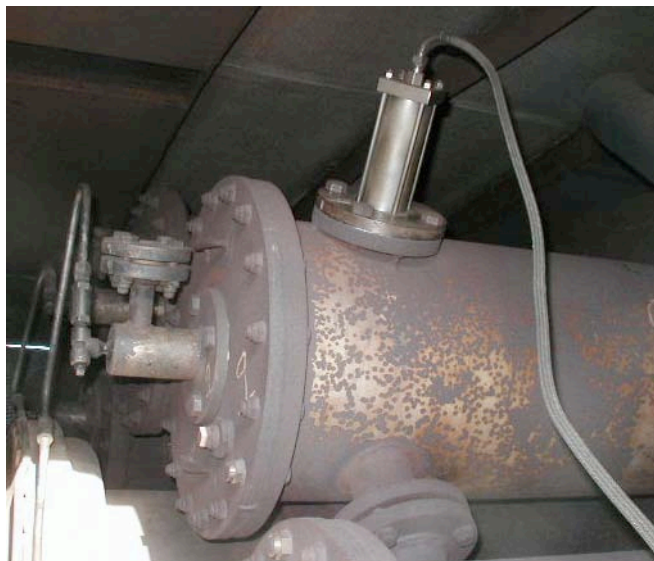
Fig. 1: Typical MS5001 Combustion Chamber with fuel nozzle
