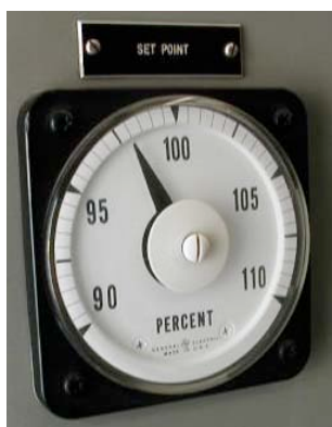
Fig. 5: Digital Setpoint Meter showing 98% “called for” speed.
