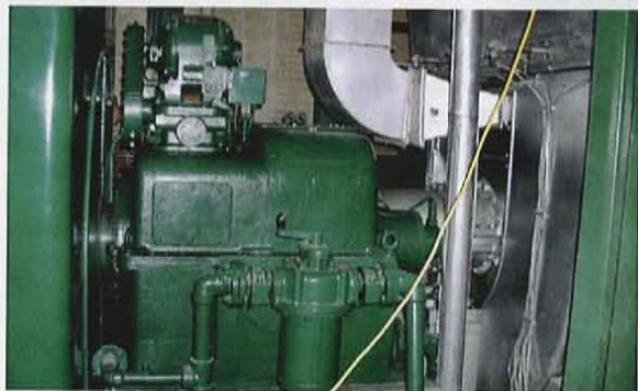
2. Turning-gear mechanism is mounted on top of the speed reduction gear (above)
