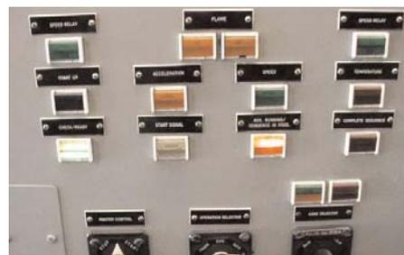
Figure 3: Panel lights (speed relays, flame detection, fuel controls)
